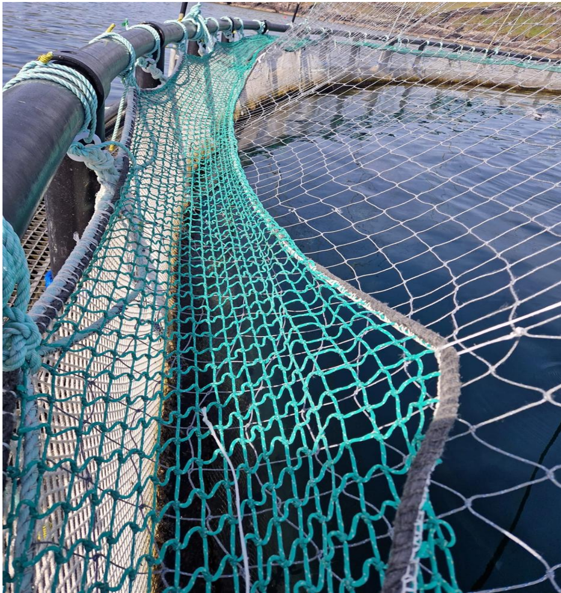
Figure 21. Seal ingress prevention protection netting at Deenish site
